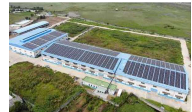
Solar panel on rooftop
