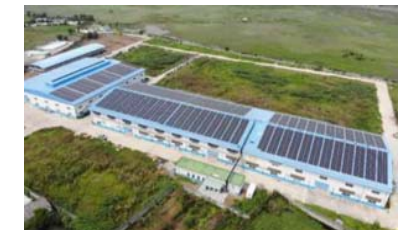
Solar panel on rooftop
