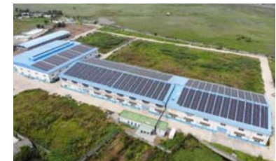
Solar panel on rooftop
