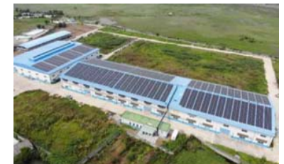
Solar panel on rooftop
