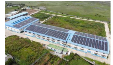
Solar panel on rooftop
