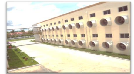
Evaporative Cooling Pad system
